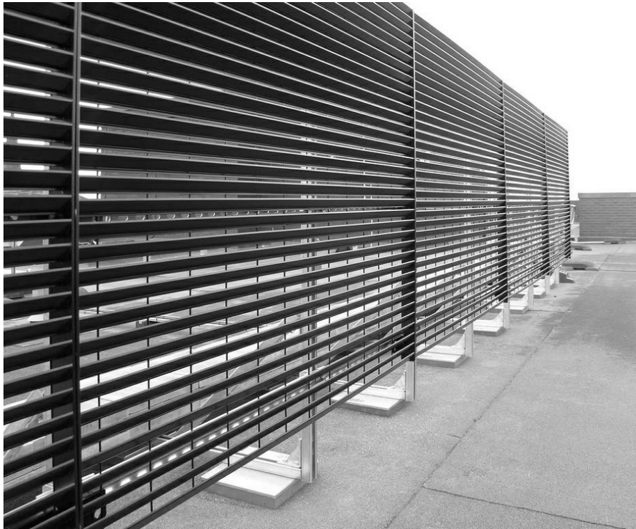
BLACK POWDERCOATED ALUMINIUM LOUVRE SCREEN
