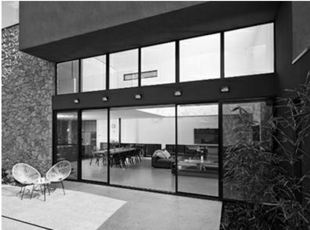
BLACK POWDERCOATED ALUMINIUM FRAMED GLAZING
